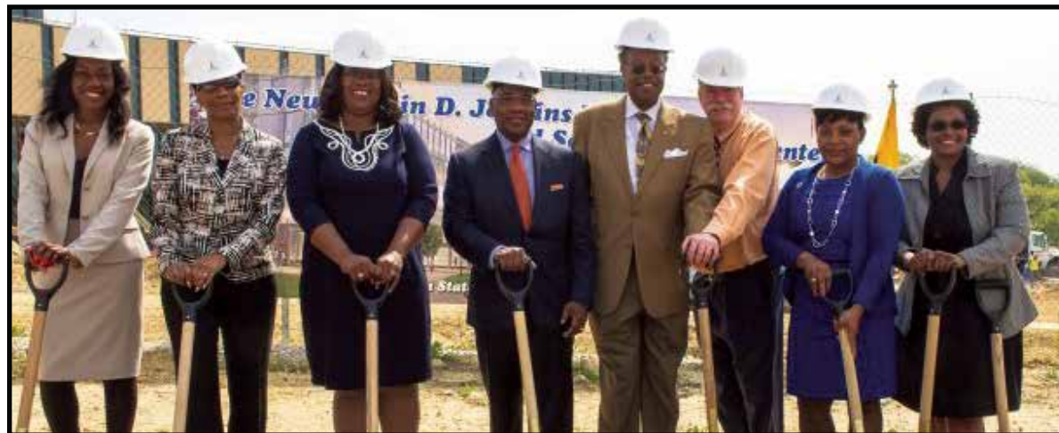
Community leaders and politicians joined Morgan State University staff and faculty to break ground on the HOK-designed Martin D. Jenkins Behavioral and Social Sciences Center (BSSC) in Baltimore.
