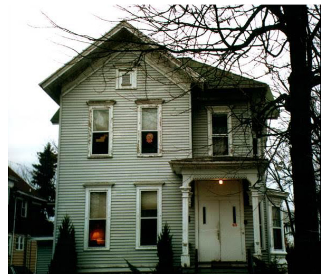
Courtesy Photo - 1980 Emergency Shelter Building
