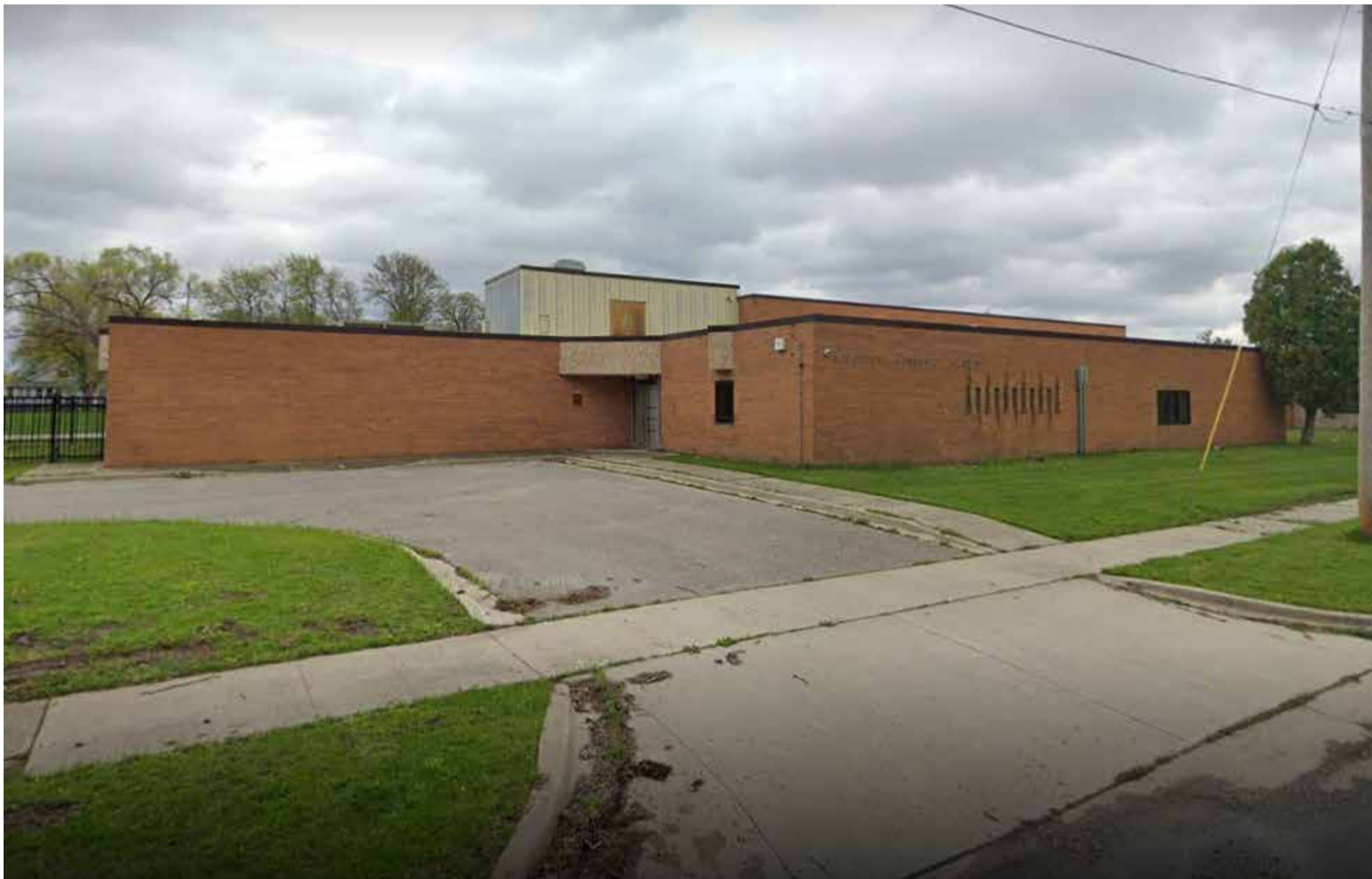
FORMER HOUGHTON ELEMENTARY SCHOOL
