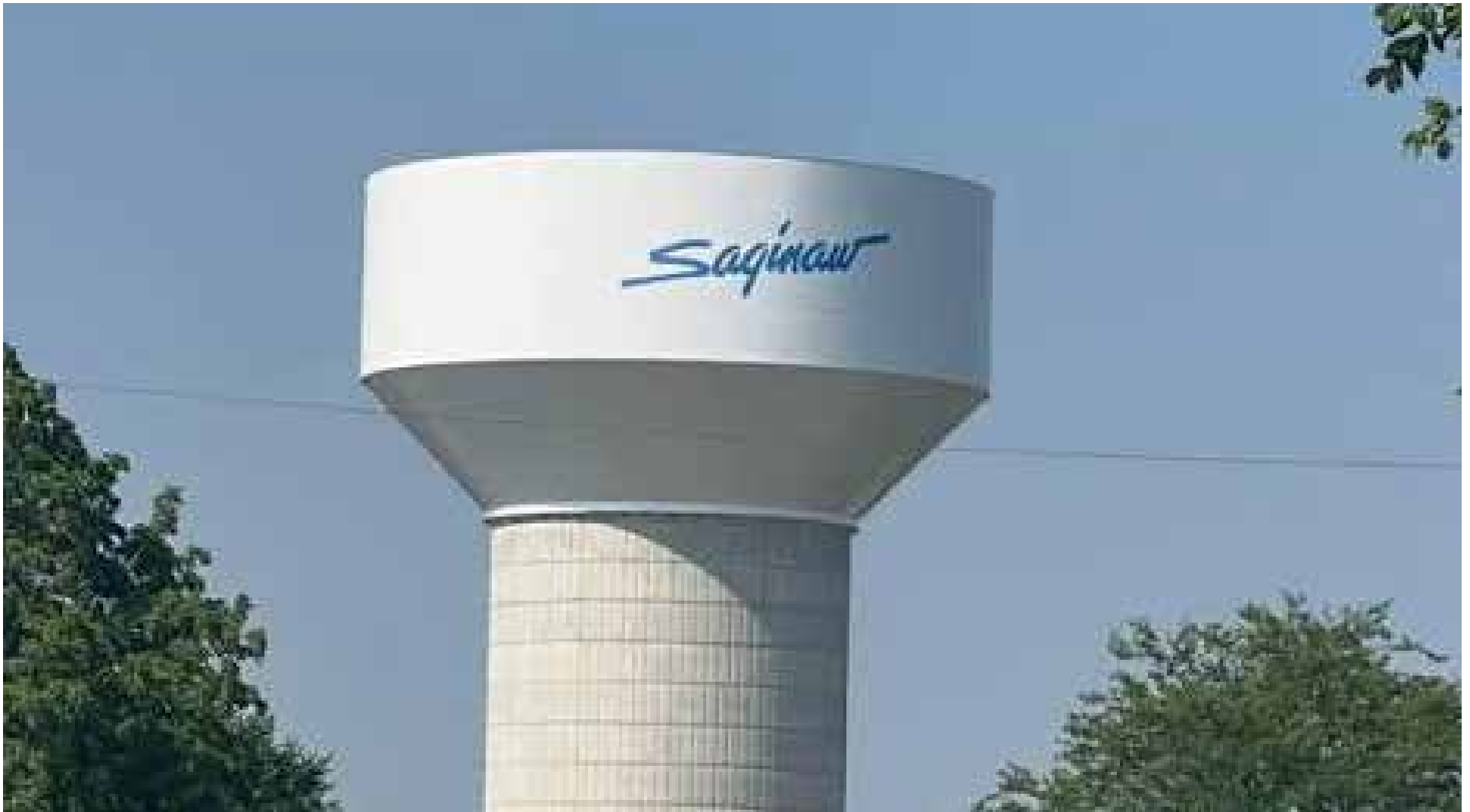
SAGINAW WILL HOLD A PUBLIC RIBBON-CUTTING CEREMONY JULY 17 FOR ITS NEW 3-MILLION-GALLON MUNICIPAL WATER TOWER AT 702 WEBBER ST. THE 160-FOOT-TALL, $18.1 MILLION STRUCTURE IS DESIGNED TO IMPROVE WATER RELIABILITY FOR MORE THAN 150,000 REGIONAL CUSTOMERS.
