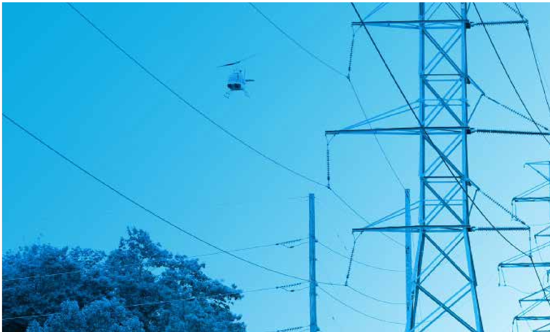
MICHIGAN ELECTRIC TRANSMISSION COMPANY IS SEEKING COMMUNITY FEEDBACK ON THE COPPERTON PROJECTS, A MAJOR EXPANSION OF MICHIGAN'S HIGH-VOLTAGE TRANSMISSION NETWORK THAT INCLUDES PROPOSED LINES THROUGH MIDLAND COUNTY. (PHOTO | ITC HOLDINGS)
