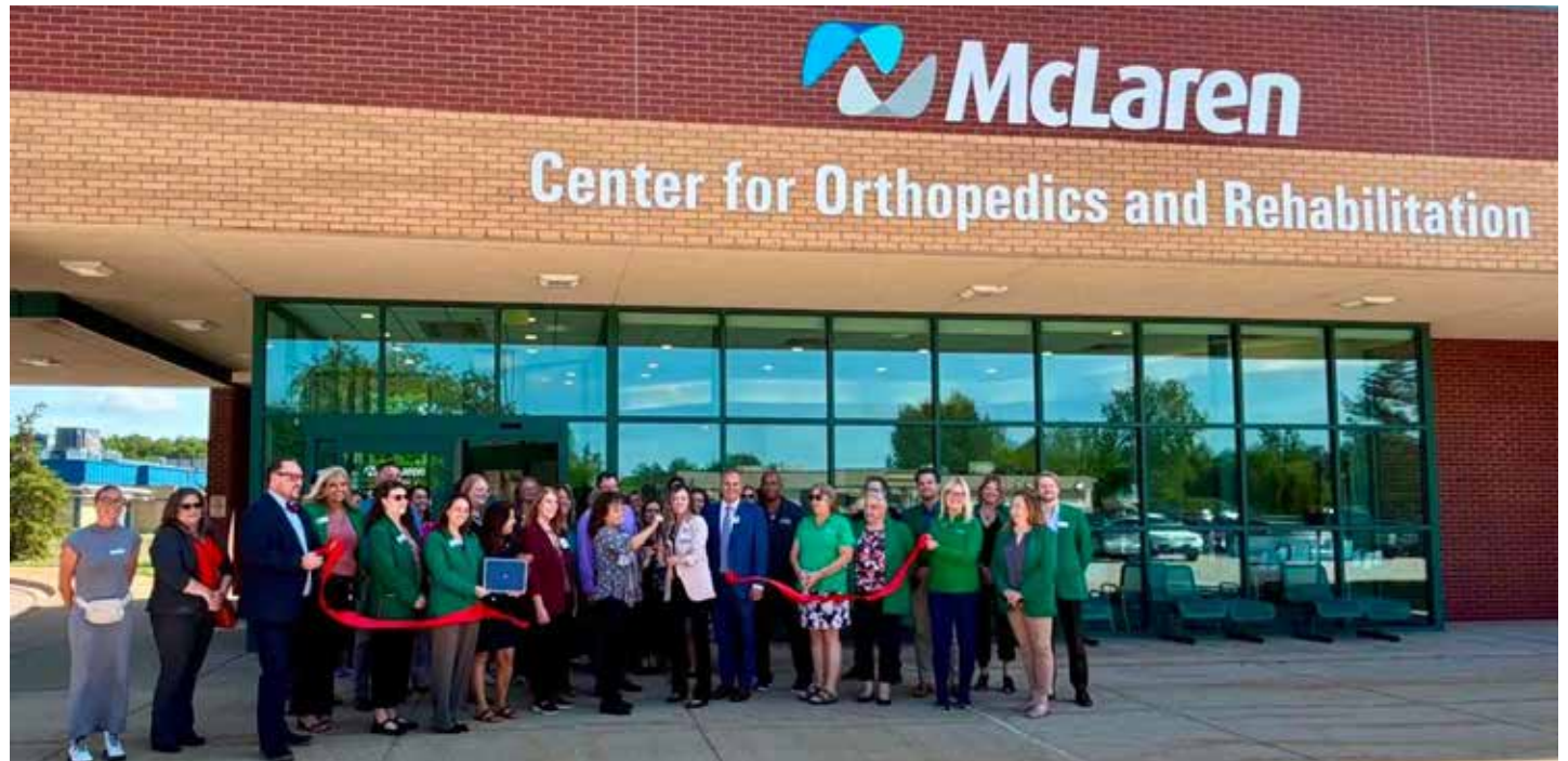
MCLAREN BAY REGION HAS OPENED THE MCLAREN BAY WEST CENTER FOR ORTHOPEDICS AND REHABILITATION, THE FIRST MAJOR COMPLETED PORTION OF ITS $53.6 MILLION REDEVELOPMENT OF THE WEST CAMPUS. (PHOTO | MCLAREN HEALTH CARE)
