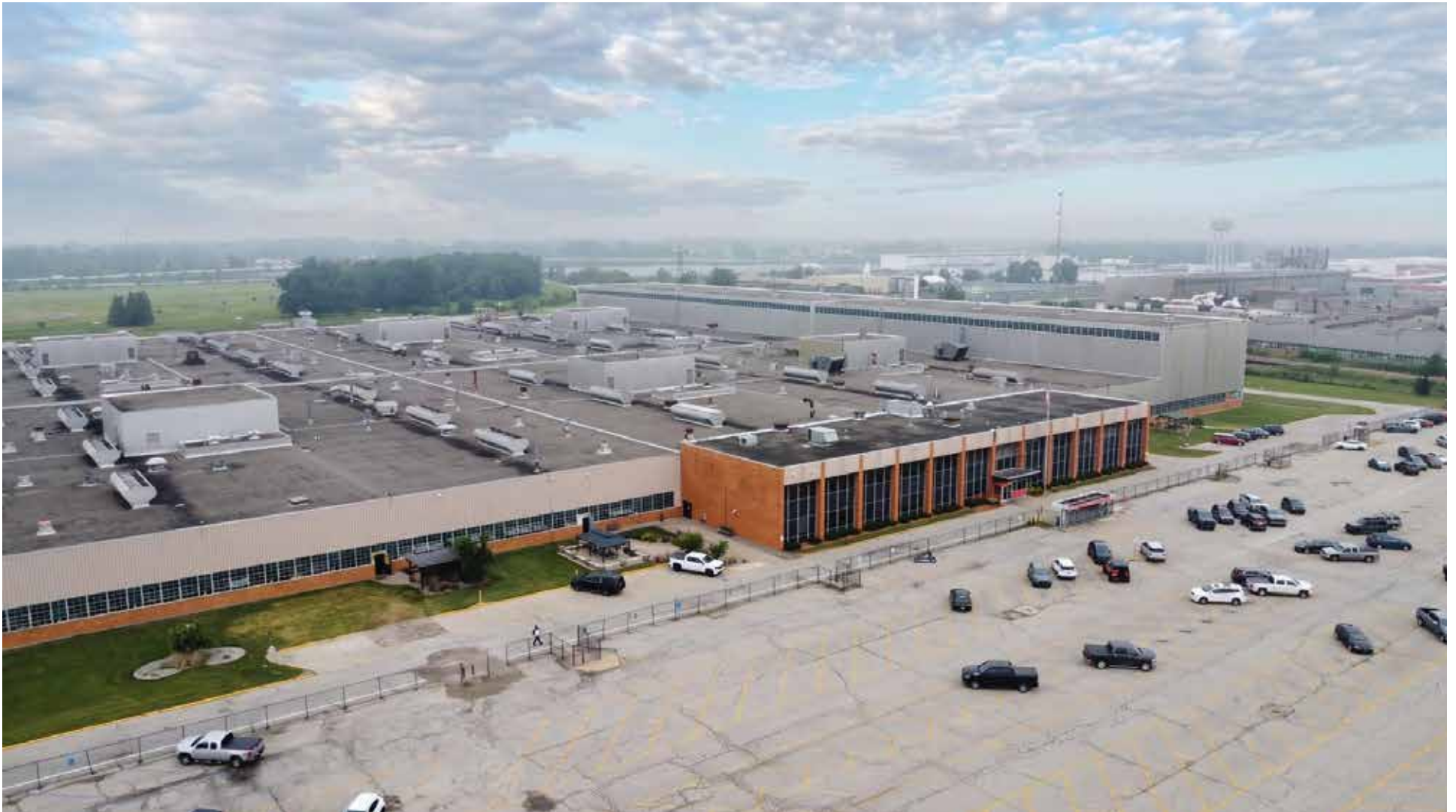
AN AERIAL VIEW OF PLANT 6 AT THE SAGINAW INDUSTRIAL CAMPUS ON EAST HOLLAND ROAD. PHOENIX INVESTORS HAS ACQUIRED APPROXIMATELY 1.8 MILLION SQUARE FEET ACROSS THREE BUILDINGS WHILE NEXTEER AUTOMOTIVE CONTINUES MANUFACTURING OPERATIONS THROUGH A LEASE-BACK ARRANGEMENT. (PHOTO | PHOENIX INVESTORS)
