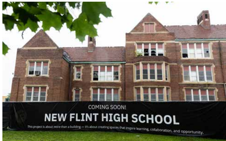
THE FORMER FLINT CENTRAL HIGH SCHOOL STANDS BEHIND A "COMING SOON! NEW FLINT HIGH SCHOOL" BANNER AS DEMOLITION BEGINS TO CLEAR THE SITE FOR A NEW CAMPUS. (PHOTO | FLINT COMMUNITY SCHOOLS)
